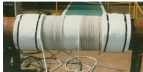
Induction coil for preheating and annealing
