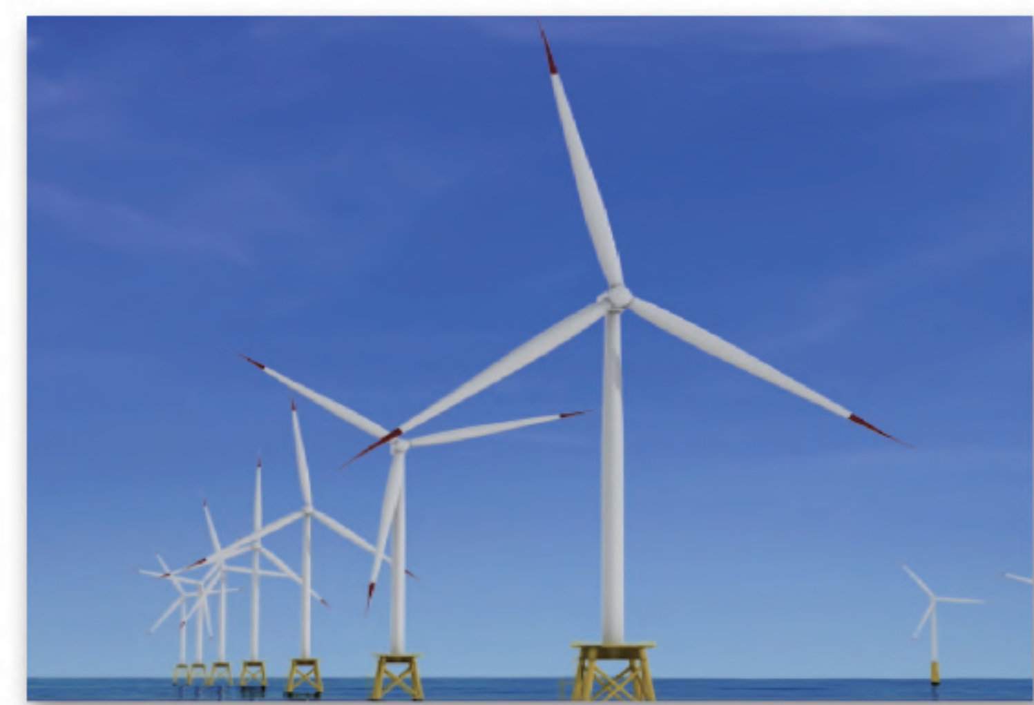
Offshore wind farm
